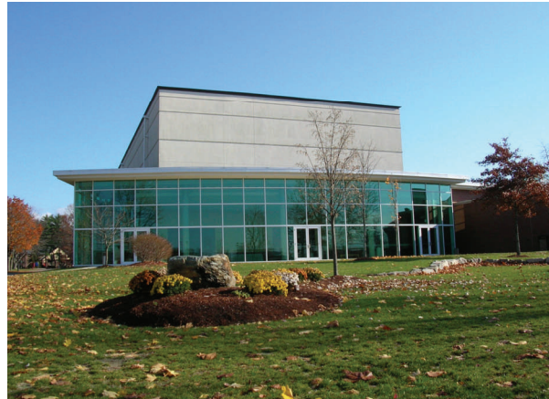
Merrimack College Rogers Center for the Performing Arts North Andover, MA
